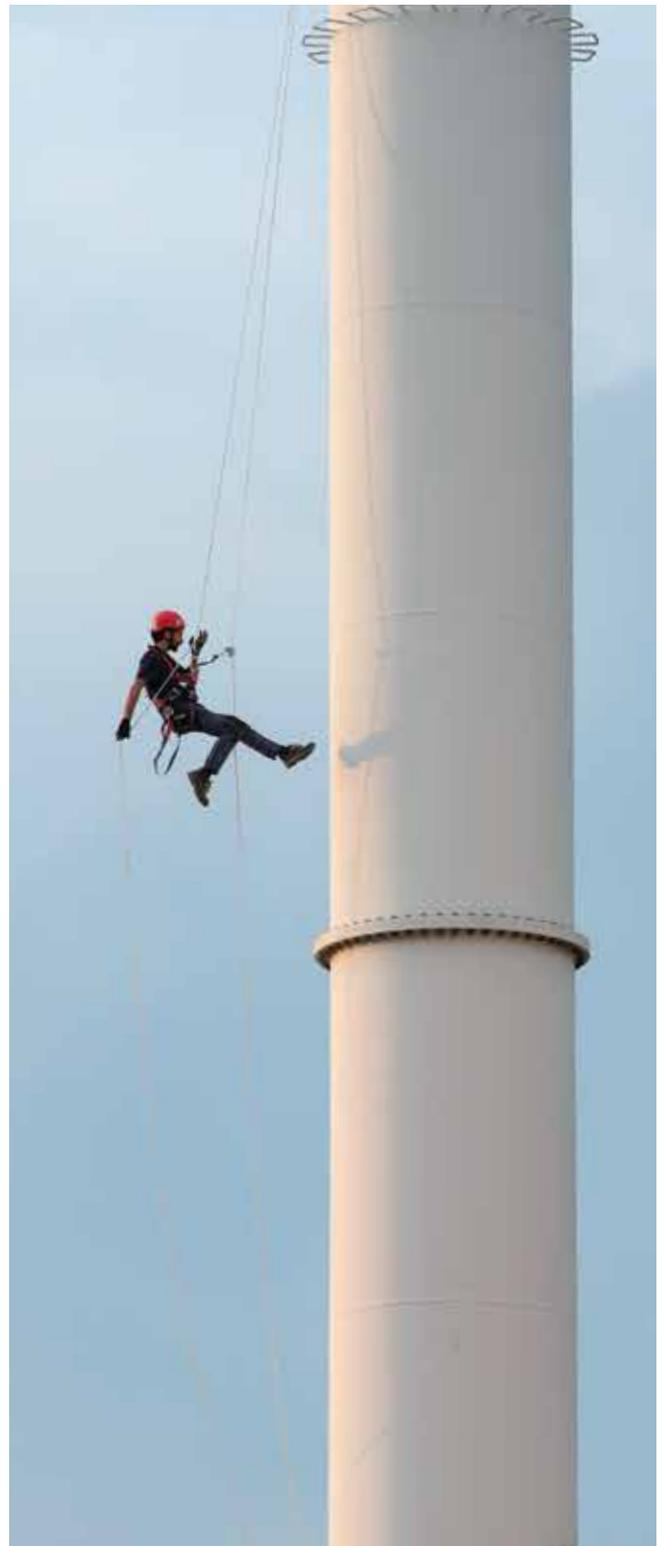
**Fig.10** - If the user is suspended and needs to climb for short distances, the worker can use a descender which also allows climbing, combined with a handled ascender and a foot loop.
